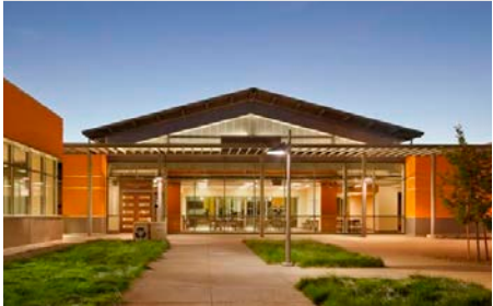
UC Davis Brewery/Winery and Food Pilot Facility Davis, CA
