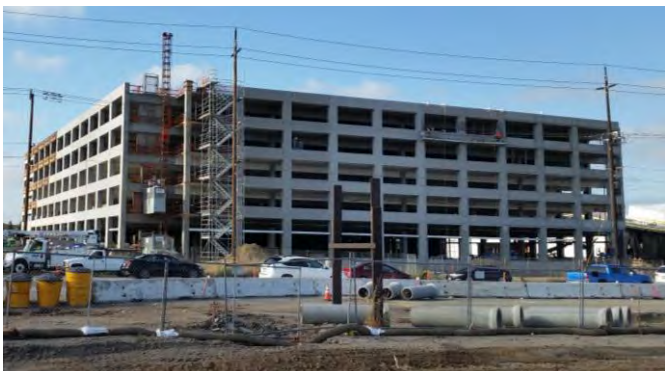
Figure 4: BART/VTA Milpitas Station Parking Structure vertical construction nearly complete.
