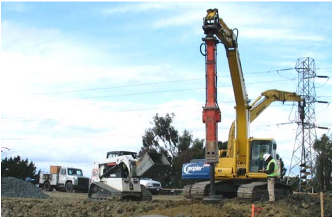
Fig.7. Typical RAP Installation Equipment
