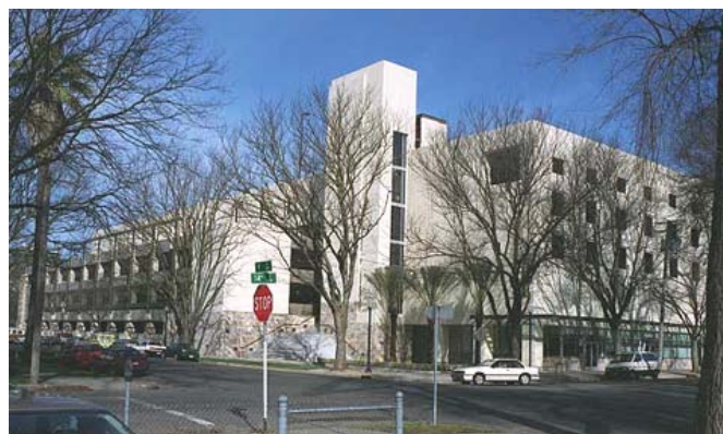
Fig.1. 1301 P Street Parking Garage, Sacramento, CA
