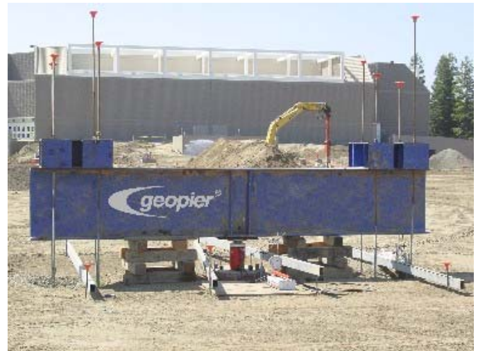
Fig.10. Section and Photo of RAP Modulus Test Set-up
